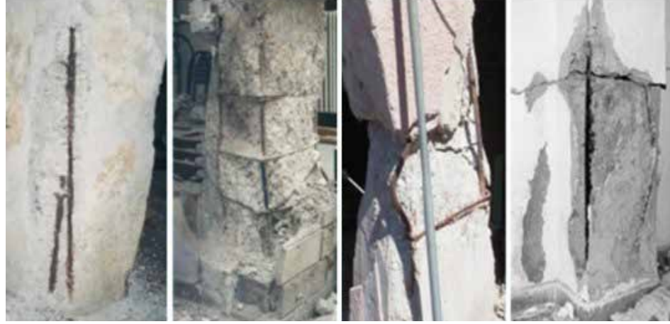
Figure 2. Corrosion of RC members damaged during the 1999 Izmit Earthquake in Turkey.
